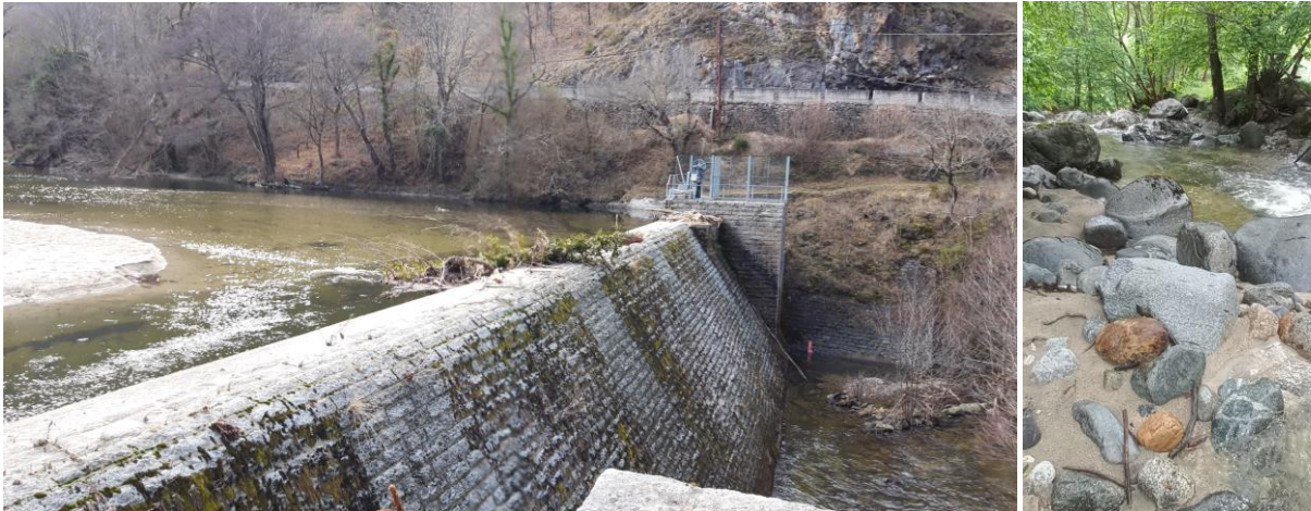
Figure 1 : Gesse water intake (GU Aude amont, 2020). After the flood of January 2020, sand deposits are present in the reservoir and in the river.
